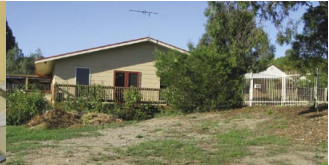
Site of the overnight cottage respite extension.
